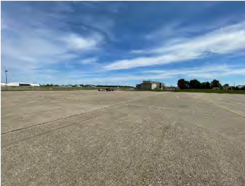
Project 14. Construct CRF Engine Storage (DCFT192002): View of paved area (proposed construction area) from Building 1 looking northeast. (Photo credit: T. Kuroiwa-Bazzan, Tetra Tech, 5/14/2021)
