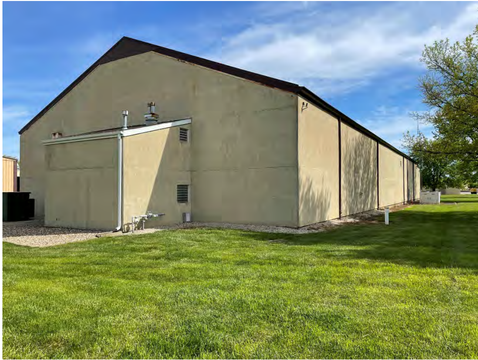
Figure 3: View Looking North.
