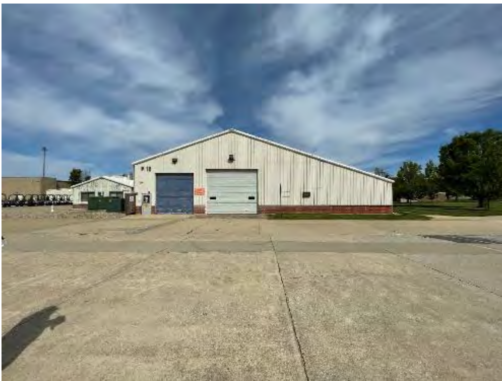
Project 5. Demolish Buildings 12 and 13 (DCFT162900): View of Building 12, looking northwest. (Photo credit: T. Kuroiwa- Bazzan, Tetra Tech, 5/14/2021)
