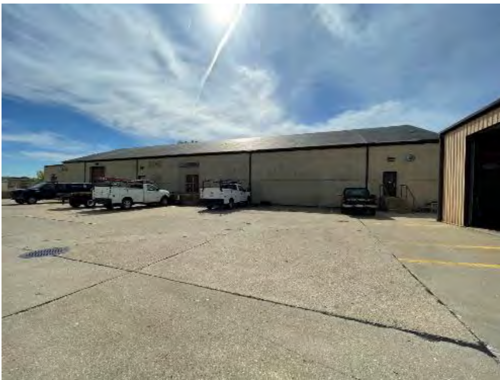
Project 19. Construct CRF Parking Lot (DCFT202008): View of Building 2, looking southeast. (Photo credit: T. Kuroiwa-Bazzan, Tetra Tech, 5/14/2021)
