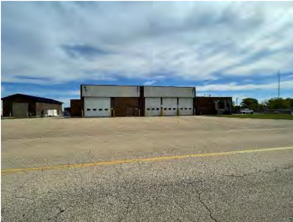
Project 3. Repair Vehicle Maintenance Facility, Building 19 (DCFT152010): View of Building 19, looking northeast. (Photo credit: T. Kuroiwa- Bazzan, Tetra Tech, 5/14/2021)
