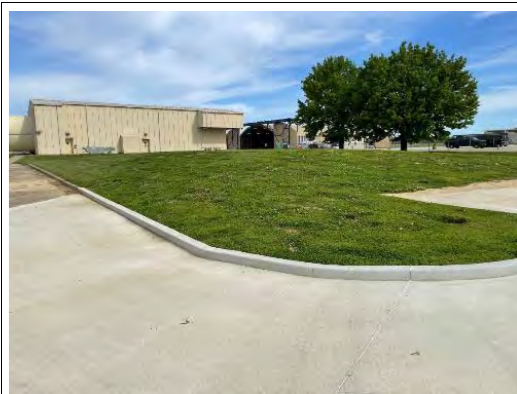
Project 13. Construct Hush House Admin Facility (DCFT192001): View of proposed construction location, looking north. (Photo credit: T. Kuroiwa-Bazzan, Tetra Tech, 5/14/2021)
