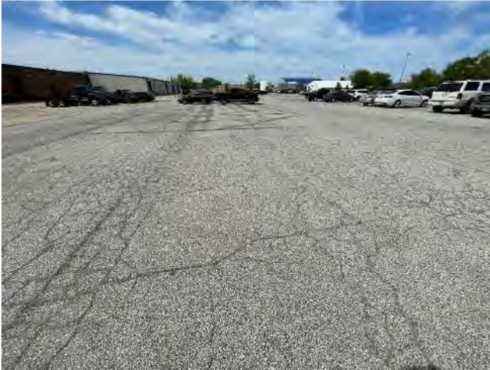
Project 9. Construct Base Civil Engineer (BCE) Complex (MILCON) (DCFT059018): View of paved area, location of proposed BCE Complex, looking southwest. (Photo credit: T. Kuroiwa- Bazzan, Tetra Tech, 5/14/2021)
