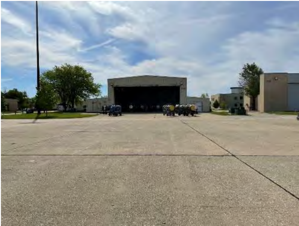
Project 1. Repair Central Repair Facility (CRF), Building 17 (DCFT102008): View of front of Building 17, looking southwest. (Photo credit: T. Kuroiwa-Bazzan, Tetra Tech, 5/14/2021)
