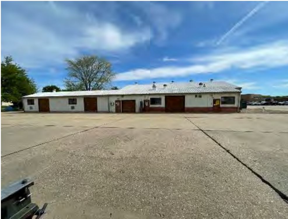
Project 5. Demolish Buildings 12 and 13 (DCFT16290): View of Building 13, looking northeast. (Photo credit: T. Kuroiwa-Bazzan, Tetra Tech, 5/14/2021)
