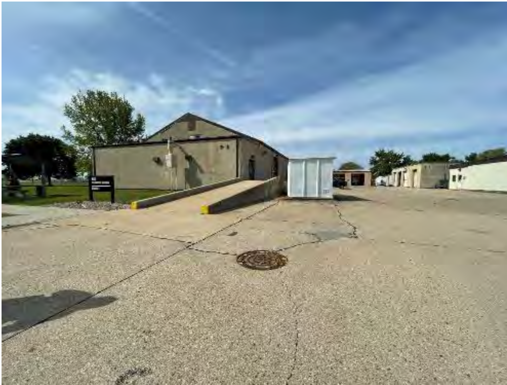
Project 19. Construct CRF Parking Lot (DCFT202008): View of Buildings 2, 3, and 45, looking southwest. (Photo credit: T. Kuroiwa-Bazzan, Tetra Tech, 5/14/2021)
