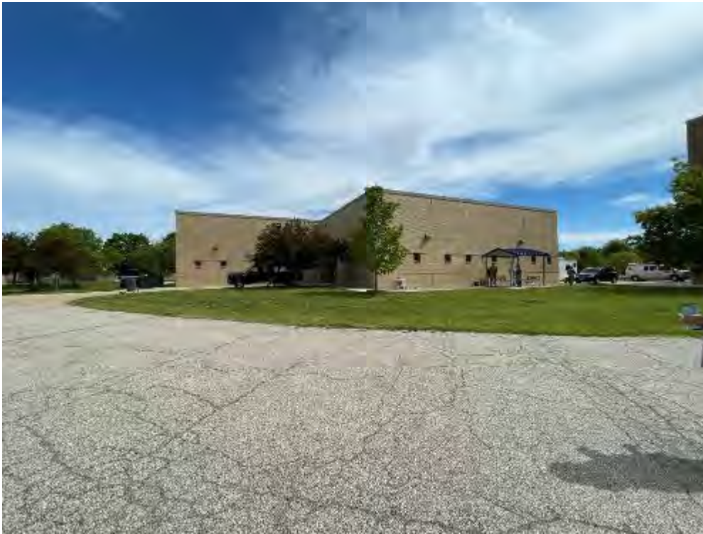
Project 10. Repair Roof, Building 46 (DCFT162014): View of Building 46, looking northeast. (Photo credit: T. Kuroiwa- Bazzan, Tetra Tech, 5/14/2021)
