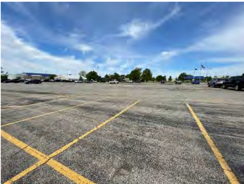
Project 9. Construct Base Civil Engineer (BCE) Complex (MILCON) (DCFT059018): View of paved area, location of proposed BCE Complex, looking south. (Photo credit: T. Kuroiwa- Bazzan, Tetra Tech, 5/14/2021)
