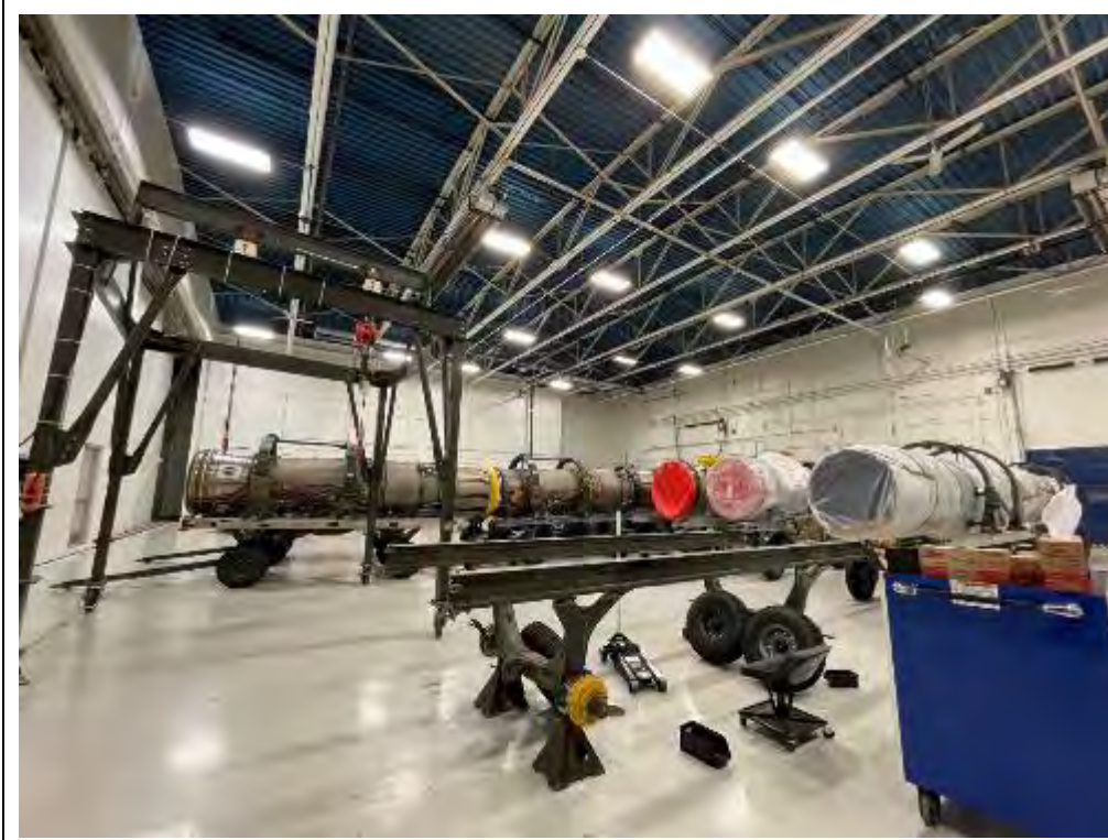
Project 12. Install Bridge Cranes / CRF Operations (DCFT182004): View of ceiling in Building 26 where cranes will be installed. (Photo credit: T. Kuroiwa-Bazzan, Tetra Tech, 5/14/2021)
