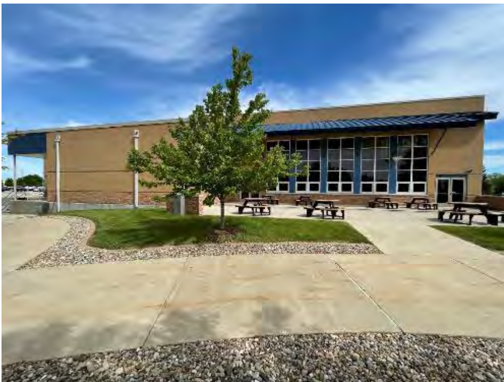
Project 8. Repair Dining Facility (DFAC) in existing Building 48 (DCFT162002): View of Building 48, looking north. (Photo credit: T. Kuroiwa-Bazzan, Tetra Tech, 5/14/2021)
