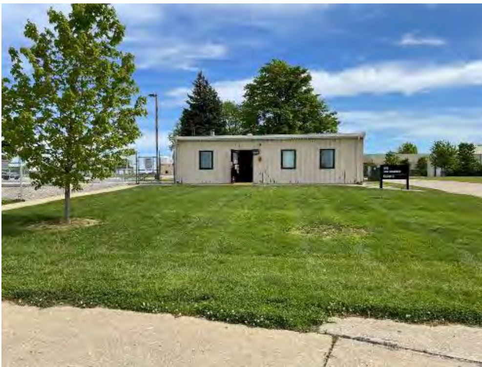
Project 15. Repair POL Facility, Building 18 (DCFT192006): View of Building 18, looking northeast. (Photo credit: T. Kuroiwa-Bazzan, Tetra Tech, 5/14/2021)
