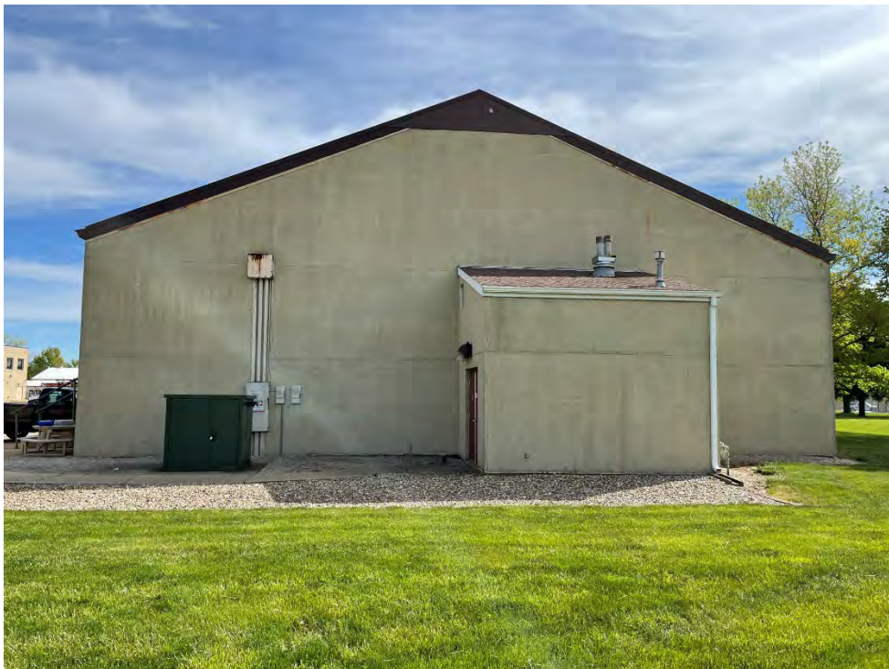
Figure 2: View Looking Northeast.
