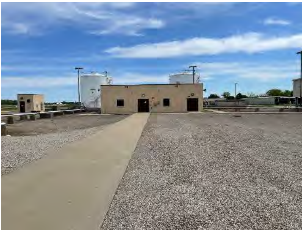
Project 18. Repair CMU Pump House and Control Room: View of POL Pump House and Control Room, looking northeast. (Photo credit: T. Kuroiwa-Bazzan, Tetra Tech, 5/14/2021)
