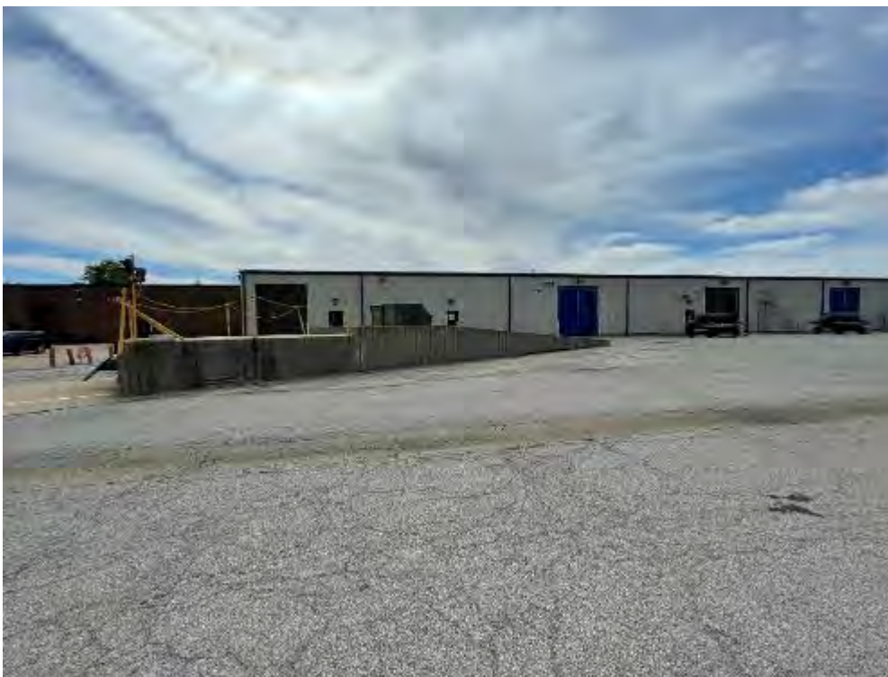
Project 6. Repair Access, Building 15 (DCFT192011): View of Building 15, looking southeast. (Photo credit: T. Kuroiwa-Bazzan, Tetra Tech, 5/14/2021)
