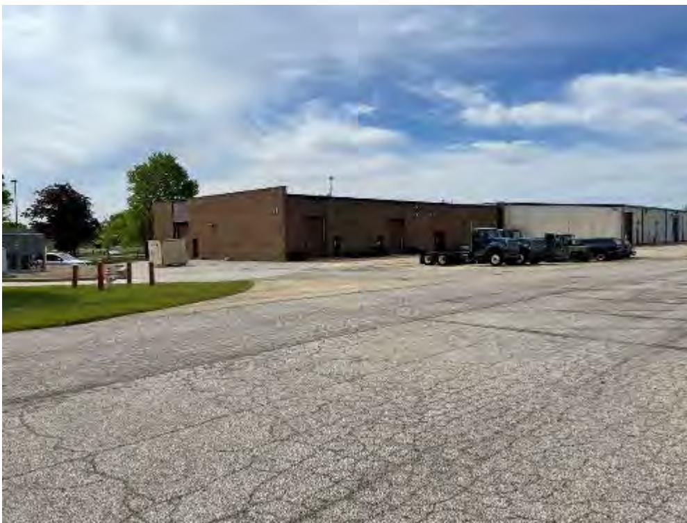
Project 11. Repair Deployment Processing, Building 23 (DCFT202001): View of Building 23, looking south. (Photo credit: T. Kuroiwa-Bazzan, Tetra Tech, 5/14/2021)
