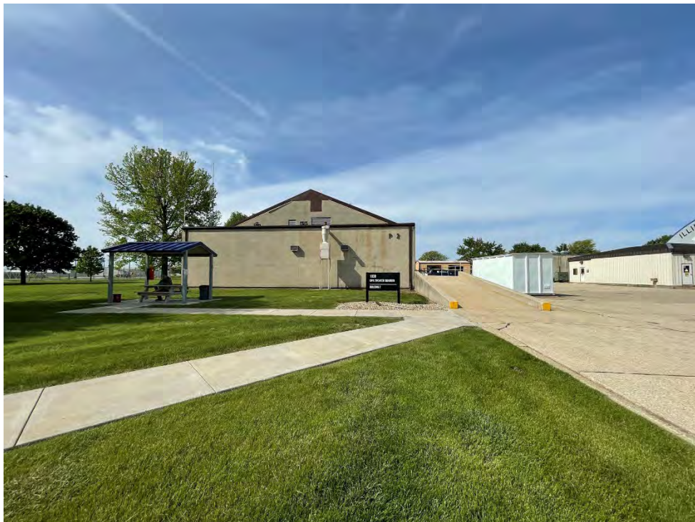
Figure 4: View Looking Southwest.
