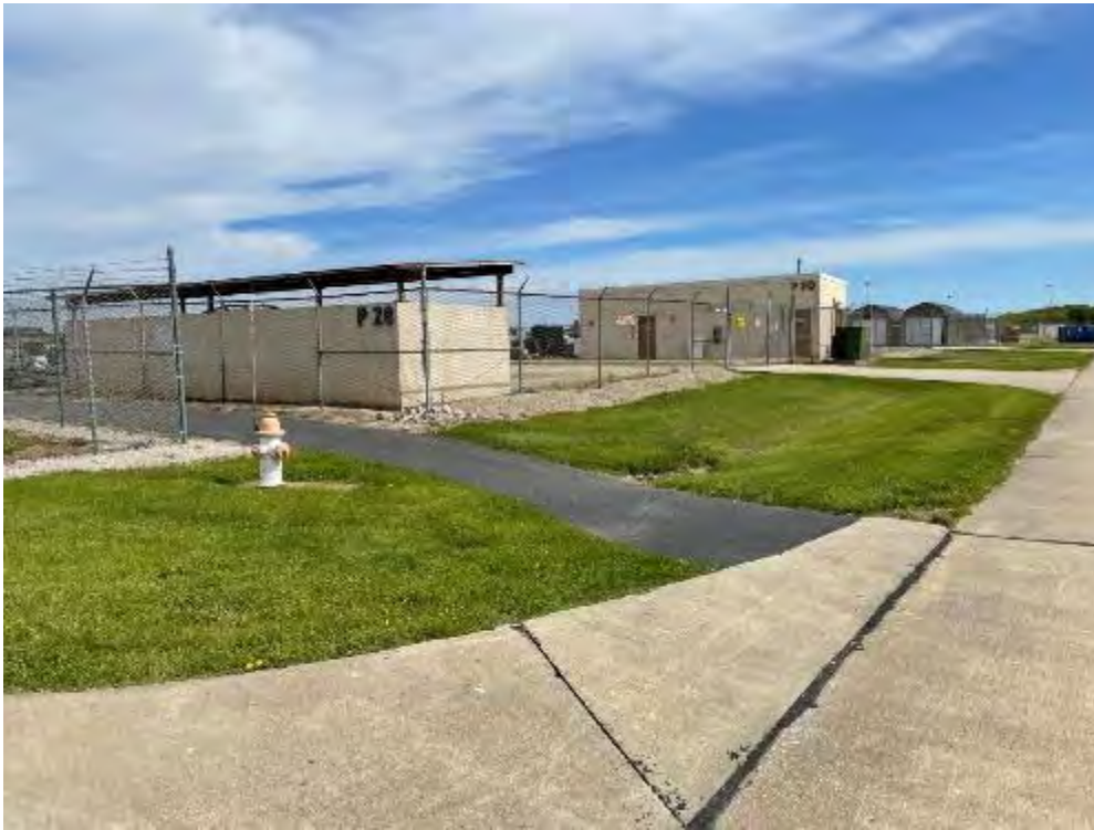
Project 16. Construct Modular Shooting Range (DCFT219001): View of proposed location of modular shooting range, looking north. (Photo credit: T. Kuroiwa-Bazzan, Tetra Tech, 5/14/2021)
